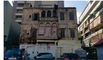
4 Local residential houses
