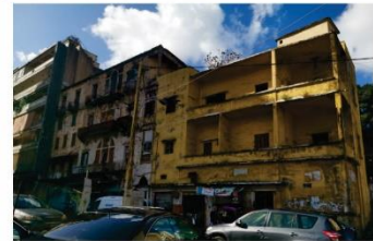
4 Local residential houses
